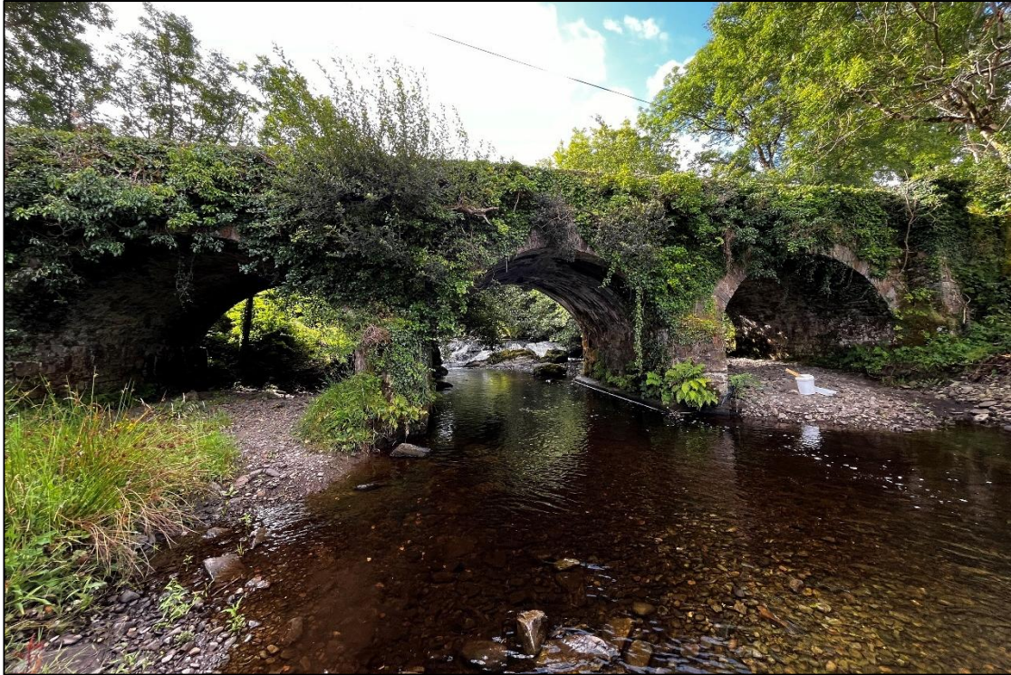
Plate 4-16. A representative picture of survey site WF 15
