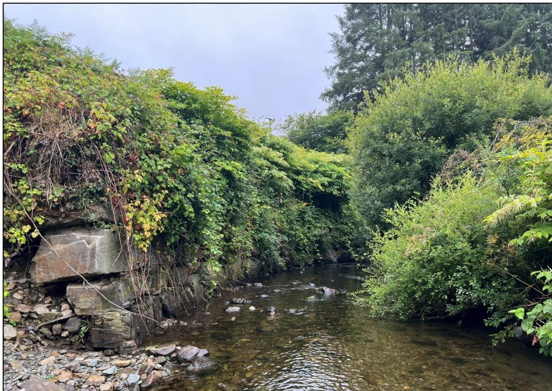
Plate 4-7. A representative picture of survey site WF 6
