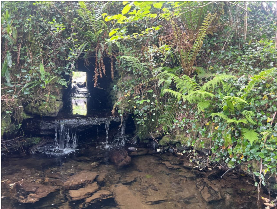
Plate 4-34. A representative picture of the under-road box culvert and raised apron at the upstream survey extent of GC 8.
